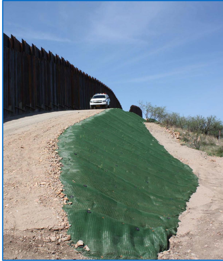
Figure 28 - Erosion Control Using High Performance Turf Reinforcing Mat
