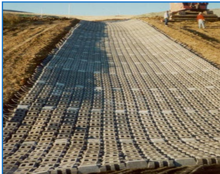
Figure 12 - Articulated Concrete Mat
