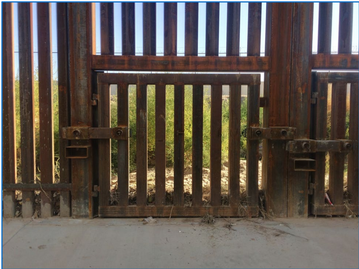
Figure 32 - Drainage Gate in Bollard Wall
