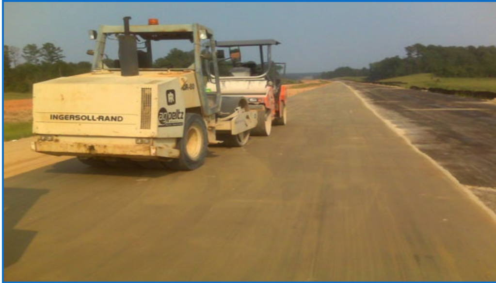
Figure 7 – Soil Stabilization with Additives
